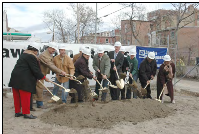
The first shovels of dirt for The Exchange were turned by Councilmember Jack Evans, ANC Commissioners, and representatives of Shaw Main Streets, Douglas Development, neighborhood churches, and civic associations.
